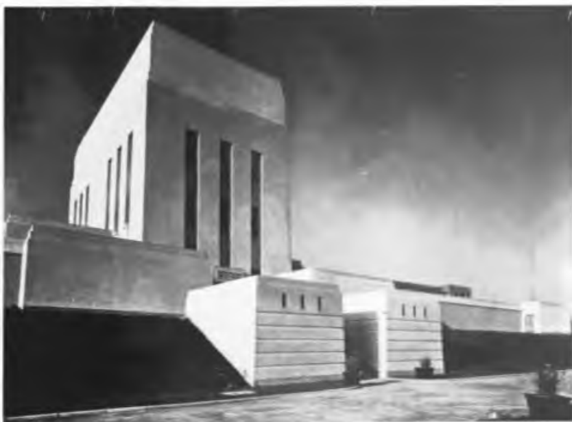
WATER WORKS, FELTHAM.
